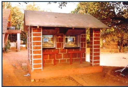
Photo 1. MIE kiosk, Kalse Village, Sindhudurg District, India
